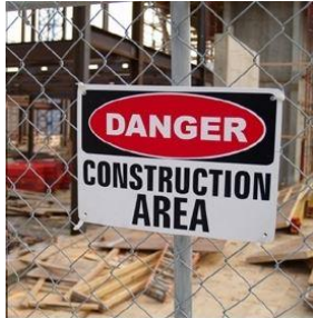
Good use of signage on fencing
