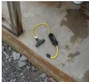
Temp GFCI cords were found throughout the work site
