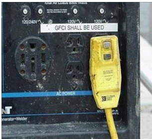
Proper use of GFCI
