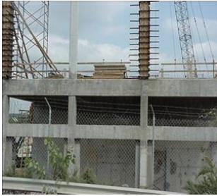
Fencing installed around perimeter of site
