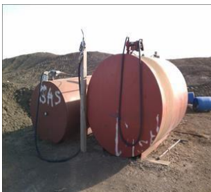
Fuel tanks are not properly labeled
