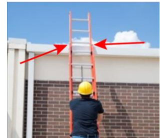
Ladder needs to be tied off
