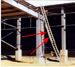
**Issue Identified** Top of ladder/side rails are not secured as needed to prevent side shift (1926.1053)
