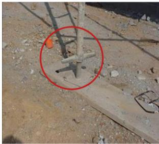
**Issue Identified**      **Scaffolds are not inspected and/or free of visible defects (1926.451)**
