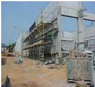
Positive Finding      Ladder or approved means are provided/used to access platform (1926.451)
