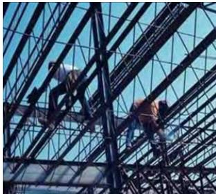
Positive Finding Perimeter safety cables are installed at all exterior/interior perimeters as soon as decking is finished (1926.760)
