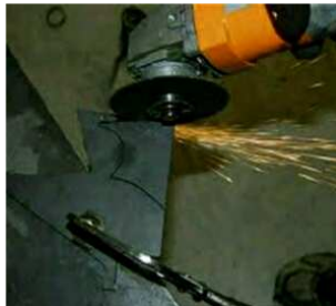
Guard missing on grinder
