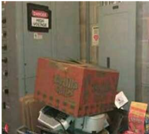
Housekeeping issue in electrical room
