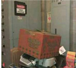
Blocked electrical panels
