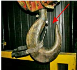
Safety latch is broken on hook in Fab shop
