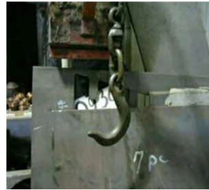
Non-approved lifting hook in Fab Shop
