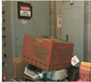
Housekeeping issue in electrical room
