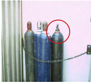
Safety cap missing
