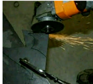
Guard missing on grinder
