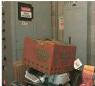
Blocked electrical panels
