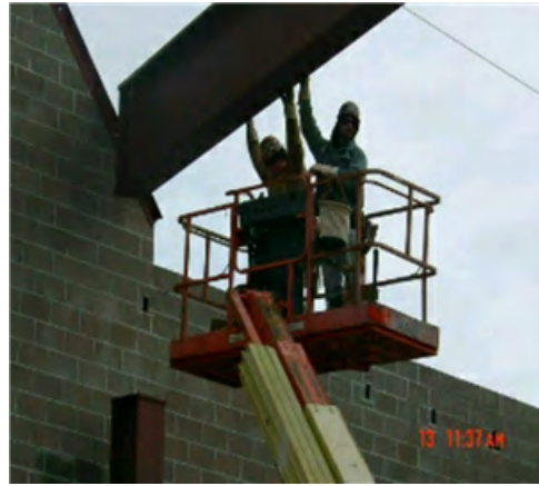
Workers have both feet on floor of lift
