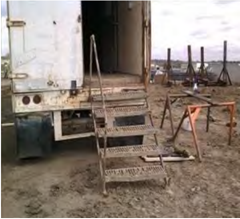
Side rails not secured
