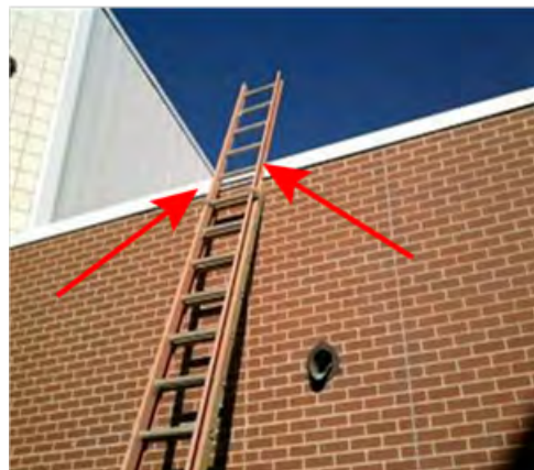
Ladder not secured to prevent side slip
