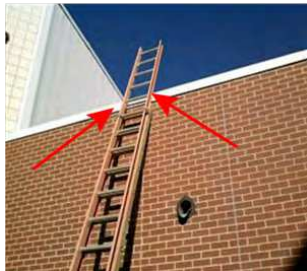
Ladder not secured to prevent side slip
