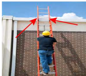
Side rails not secured
