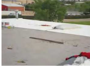
No warning line erected on north end of roof.
