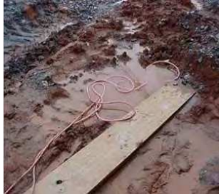
South end of project near Master storage trailer.
