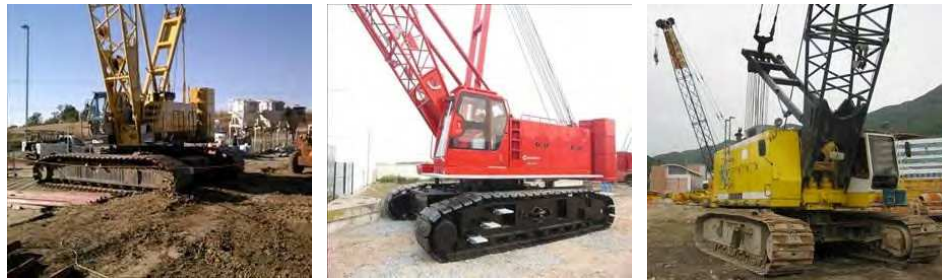
Radius guard not installed.
