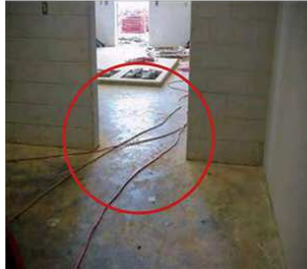
Trip hazard, cords need to be rerouted.
