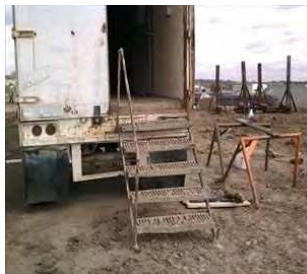
Need handrail on steps to storage trailer
