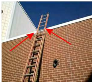
Ladder not secured to prevent side slip
