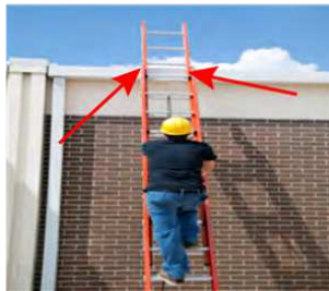
Side rails not secured
