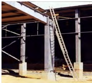
Ladder not secured to prevent side slip
