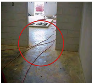
Trip hazard, cords need to be rerouted.
