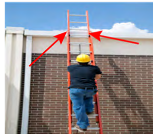
Side rails not secured
