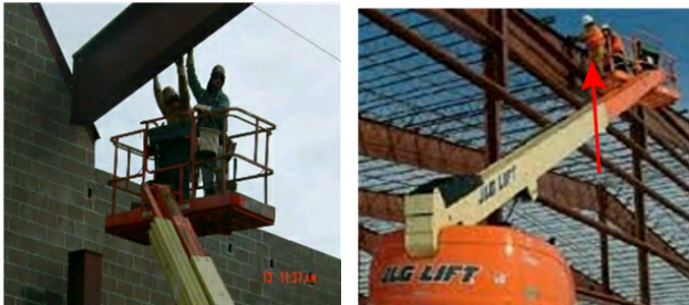
Workers have both feet on floor of lift
