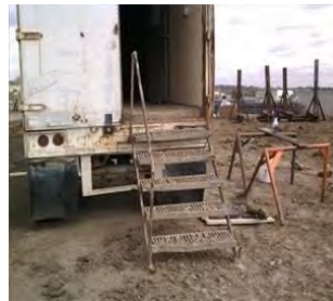
Need handrail on steps to storage trailer
